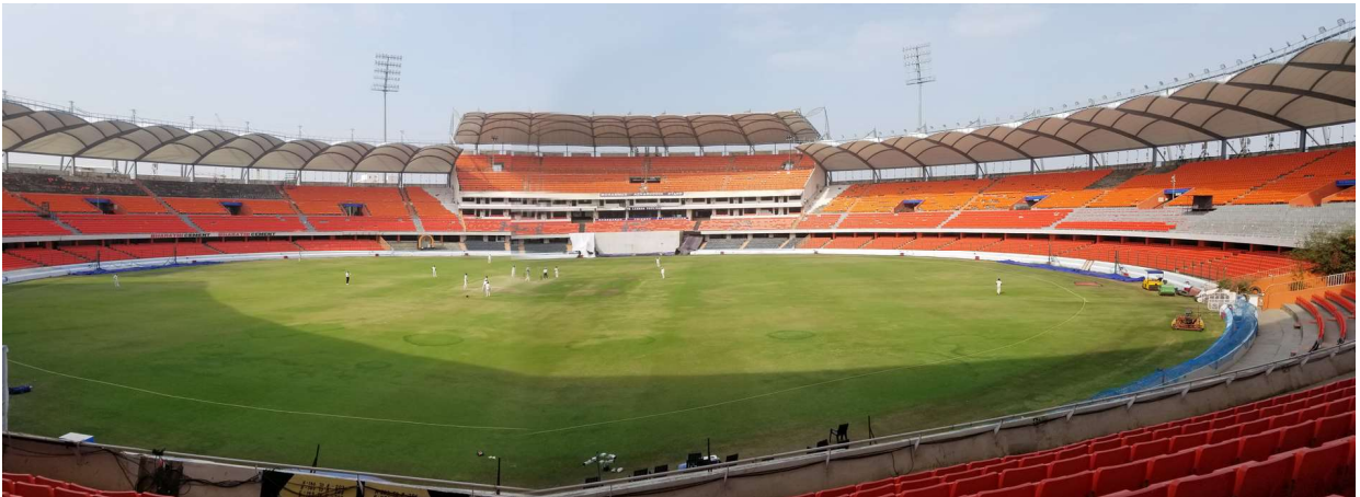
The stands are covered with tensile canopy all around.
